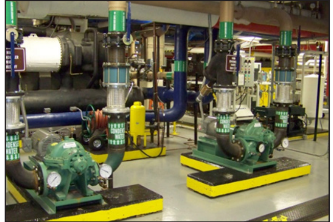
This is an example of pumps found in a hospital mechanical room. The OMEE program maintains the facility and performs preventive maintenance and repairs on these types of systems.
